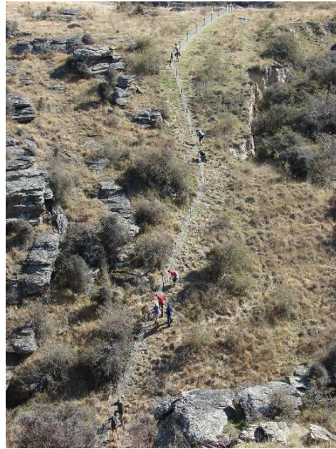
Volunteers laying rocks along part of the 1.6 km-long herbivore-proof fence to keep out rabbits and hares
